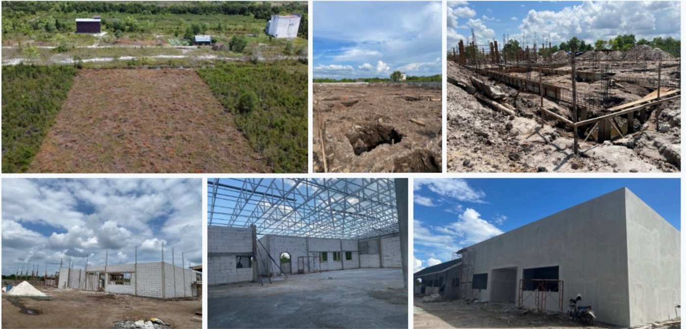
Progress of IGI Mission Center Construction
